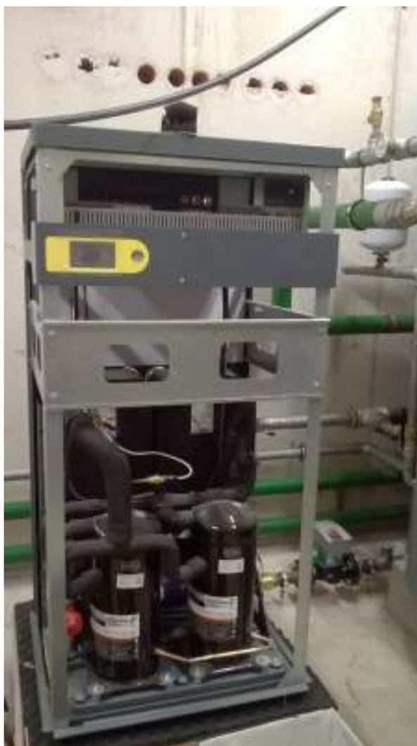
**CENTRALE TECNOLOGICA – POMPA DI CALORE GEOTERMICA**
